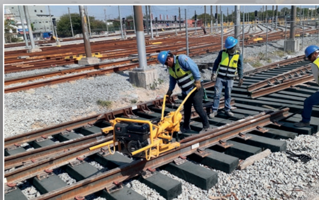
KLP® Hybrid Polymer Switch & Crossing Sleepers, Monterrey (Mexico).
